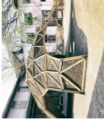
The Shell Mycelium Pavilion, India, by Yassin Areddia Designs. The fungus ate the wood and merged with it. The structure then biodegraded.
